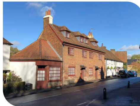
Tall brick chimneys
