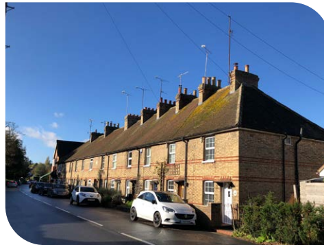
Yellow brick and clay roofs
