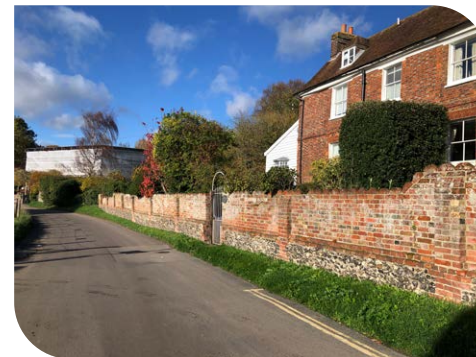
Flemish bond brickwork
